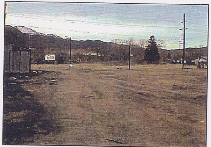
Example of "Deterioration of site or other improvements;s, and; Inadequate public improvements" factors a and j.
