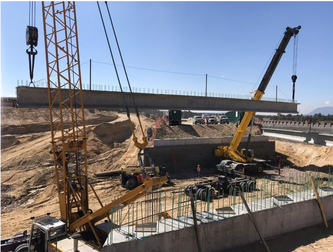
Two cranes work simultaneously to lift the girders into place.
