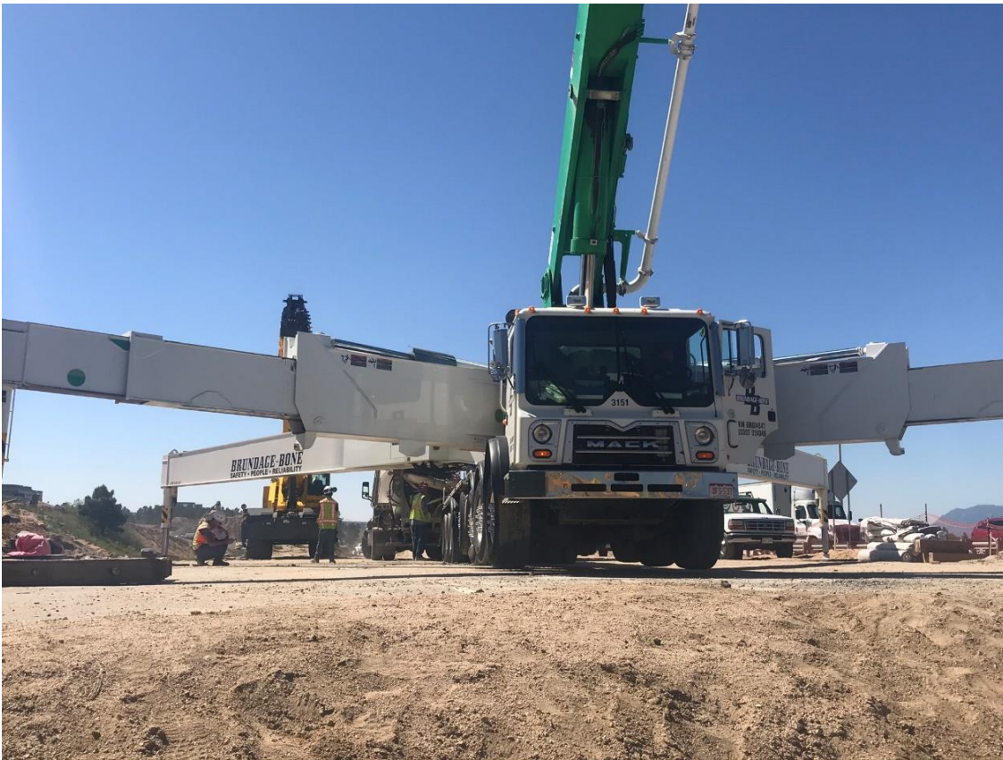
Concrete pump truck.
