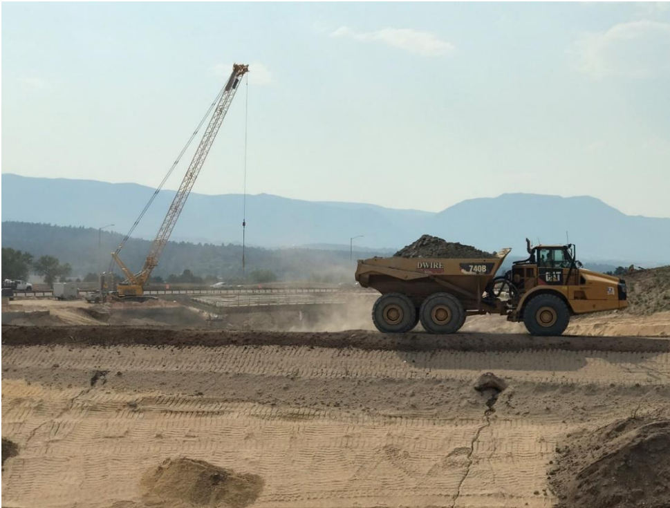
One of Dwire's 24-cubic yard trucks hauling excavated material to the future retail site in Polaris Pointe.
