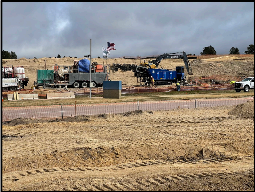
Utility Work along North Gate Boulevard
