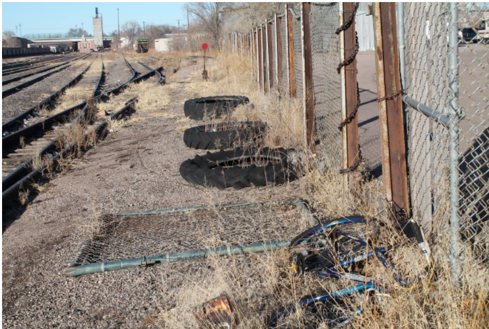
Figure 2-7 Presence of trash and debris, abandoned/inoperable equipment, potentially hazardous conditions, vagrants/vandalism/graffiti, inadequate site maintenance, non-conformance to development regulations (Photo B-29)
