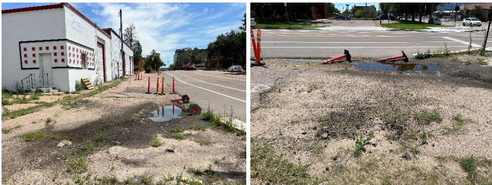
Figure 9. Evidence of Standing Water
