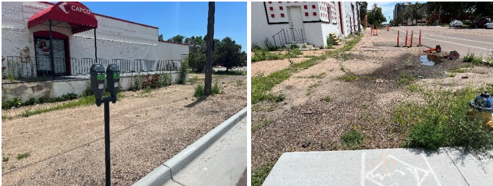
Figure 13. Lack of Sidewalks and Curb
