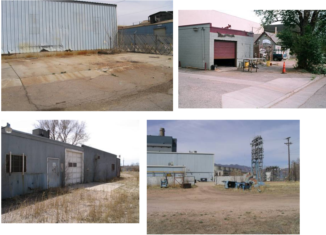
Exhibit 8: Examples of Condition E: Deterioration of Site or Other Improvements
